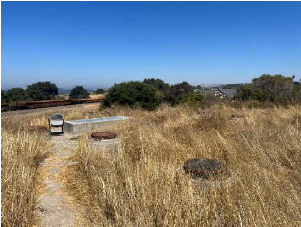
9. Storm drains on northeast portion of subject property
