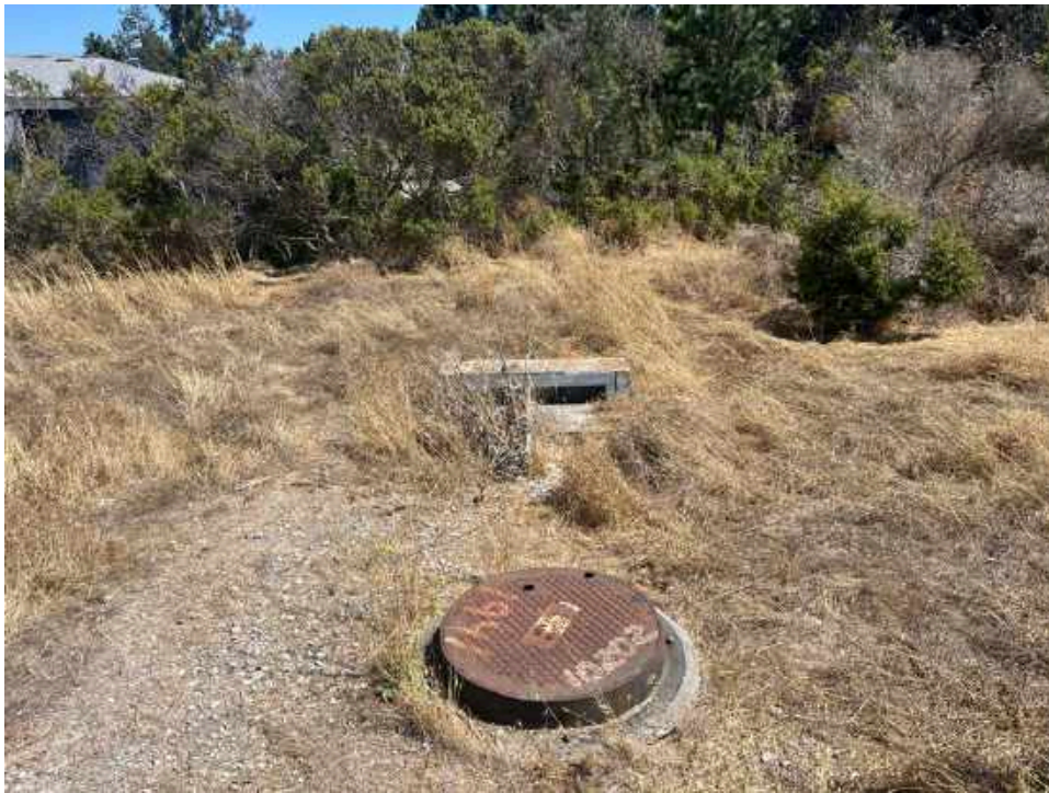
10. Storm drain on northeastern portion of subject property
