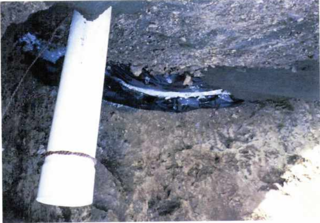
Photo No. 8 View of PVC casing and geotextile during backfilling operations
