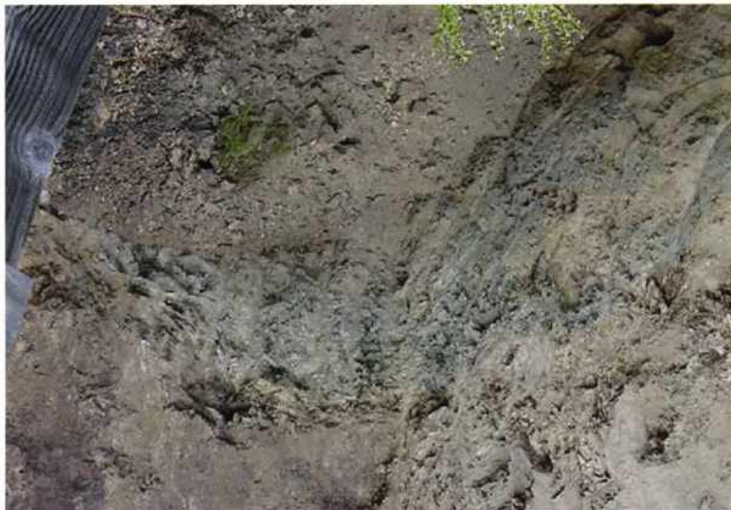
Photo No. 5 View of stained soil on north and east walls left in place in the northeast corner of the over-excavation
