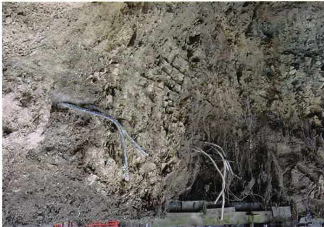
Photo No. 5 View of stained soil on north and east walls left in place in the northeast corner of the over-excavation
