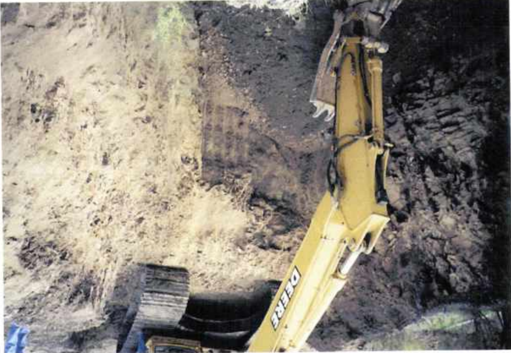
Photo No. 7 View of west wall demonstrating no staining
