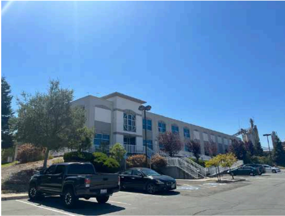
17. South adjoining commercial building
